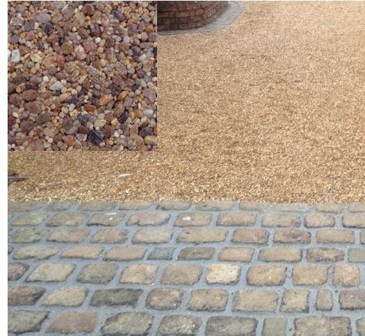
Self bonding gravel - Mocha (or similar) & Marshalls - Fairstone Cropped Granite Setts (or similar) - Court yard and parking.
